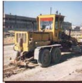
Mix treated soil to uniformity
